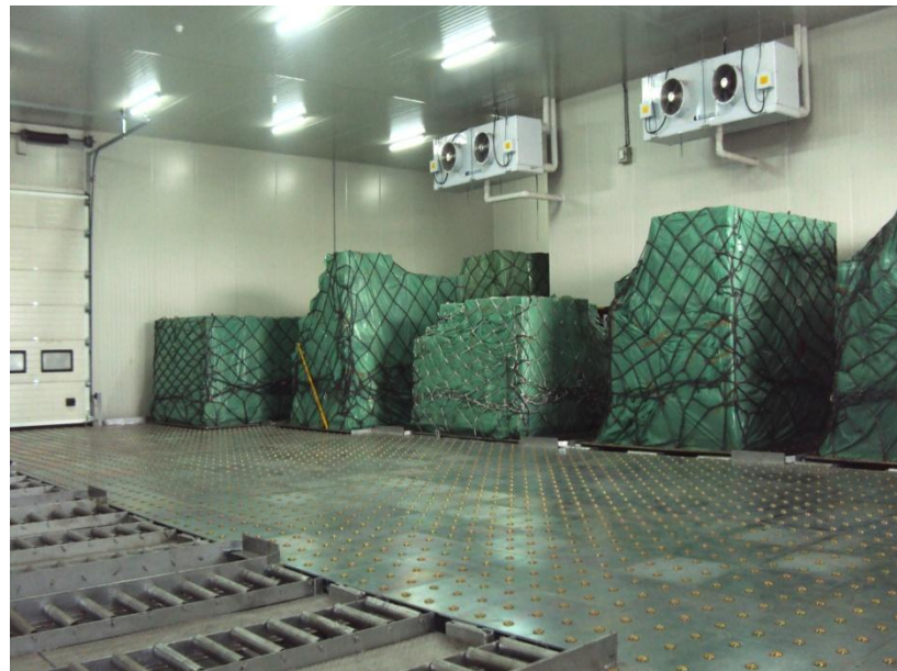
Airline Container/Pallet storage area
